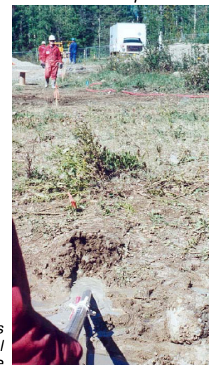
Installation of wells into horizontal fractured borehole
