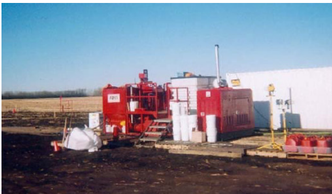
Fracture enhanced salt drainage
